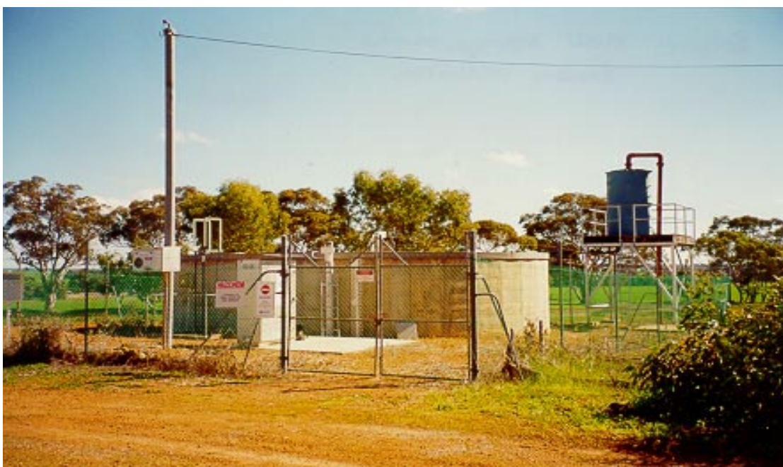
Plate 4. Bolgart town water supply storage tanks.
